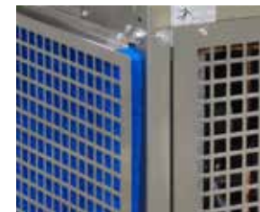
Typical Condenser Screen.
