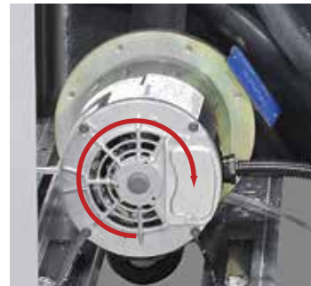
Correct shaft rotation is clockwise.
