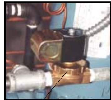
Make-up solenoid valve Figure 3.2A
