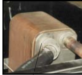
Typical evaporator
