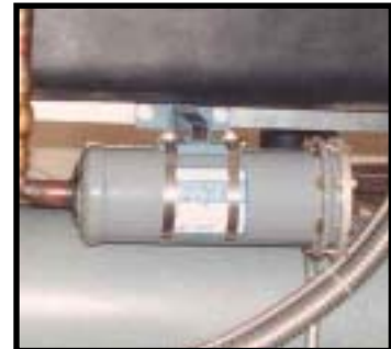
Typical filter-drier Figure 6.2D
