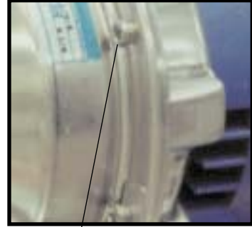
Typical pump casing bolt Figure 5.5D
