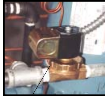
Typical water make-up solenoid valve Figure 5.4A
