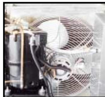
Typical air-cooled condenser
