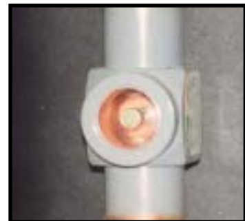
Refrigerant sight glass Figure 6.2E
