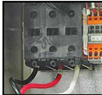
DO NOT reverse power leads at the unit's power entry to correct phase.
