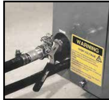
Typical drain valve installation (Shown on S-925)
