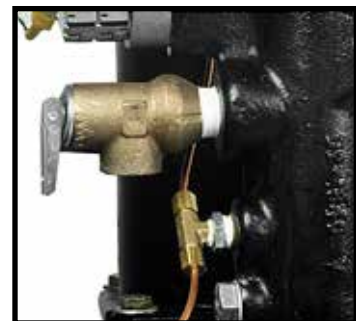
Typical pressure relief valve
