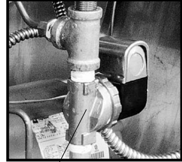
Typical cooling solenoid valve on RK units
