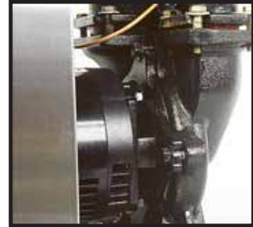
Pump casing bolts
