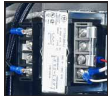
Control circuit transformer fuse Figure 2.5C
