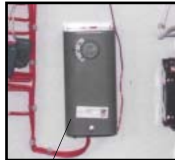
Mechanical freezestat Figure 6.1C
