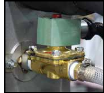
Typical Water Make-up solenoid valve
