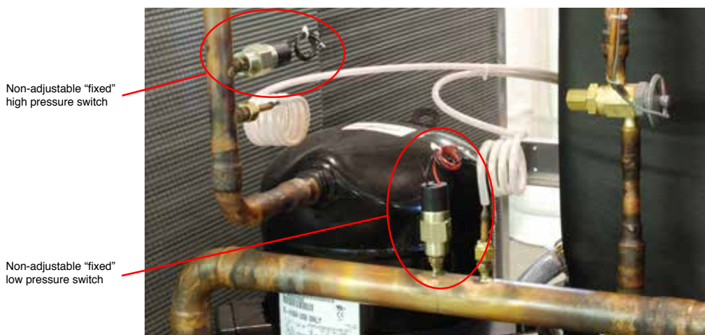
Typical placement of non-adjustable “fixed” pressure switches.
