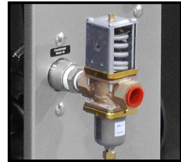
Typical water saver regulator valve.
