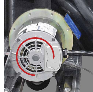
Correct shaft rotation is clockwise.
