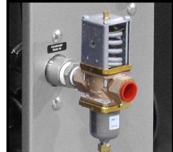
Typical water saver regulator valve.
