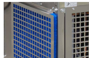
Typical Condenser Screen.
